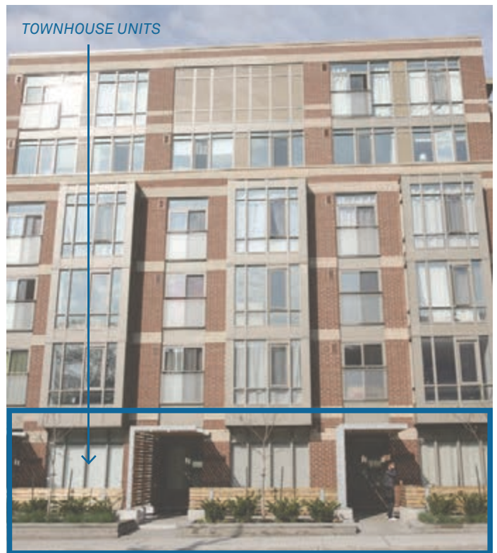
Individual townhouse units at the base of a Mid-Rise building establish privacy and provide natural light for the unit. (Image Credit: Brook McIlroy)
