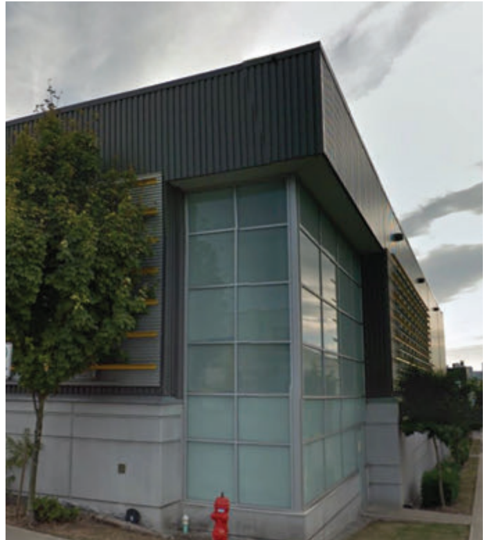
Industrial Building with generous landscape and reduced blank walls. (Image: Hallmark Poultry Processors, Google Maps)
