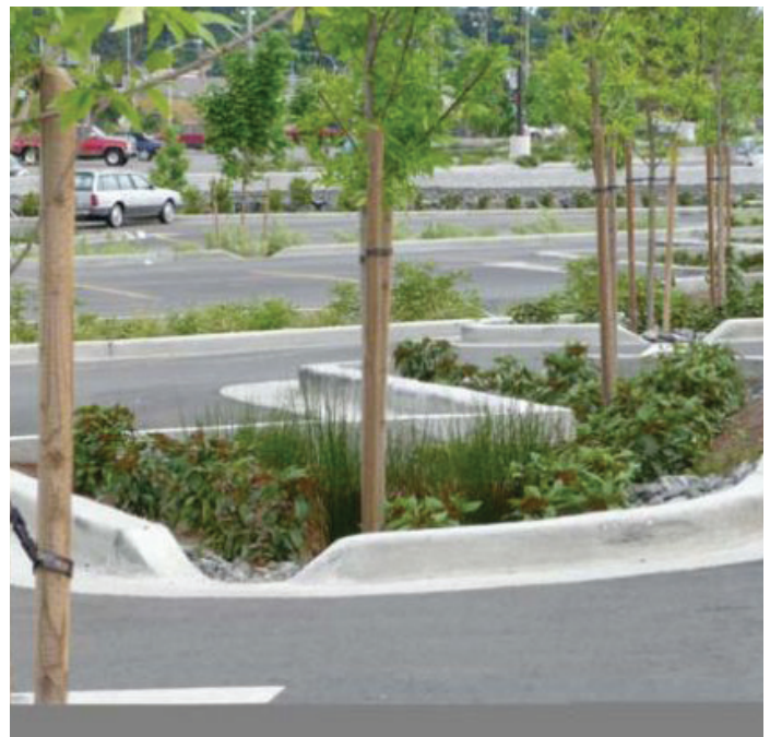
A rain garden with trees supports stormwater management. (Image Credit: Brook McIlroy).
