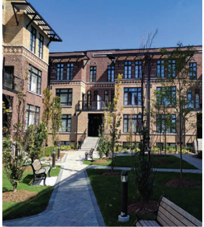
Buildings framing an internal courtyard and amenity spaces. (Image Credit: Brook McIlroy)
