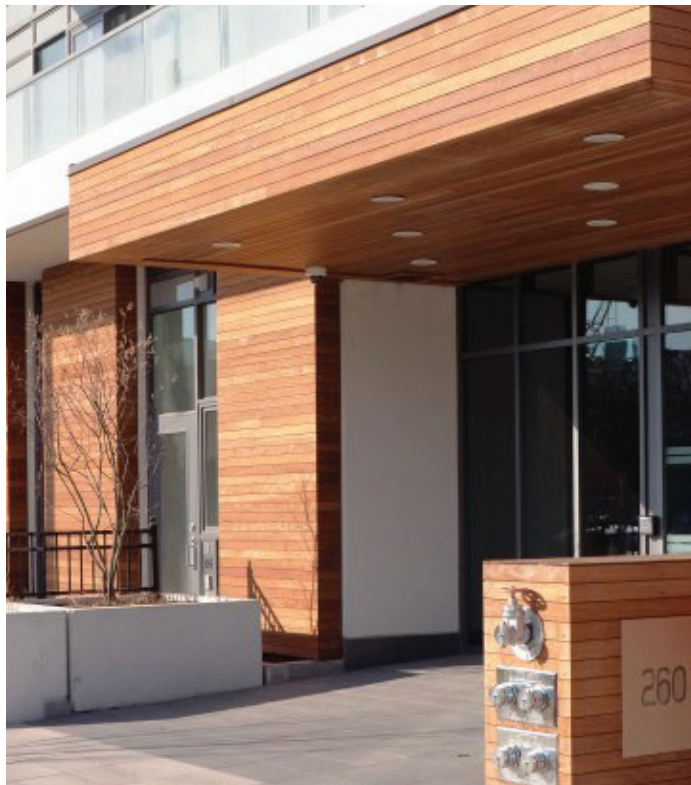
Downlighting integrated into a building entrance. (Image Credit: One Park West, Core Architects, Inc.)
