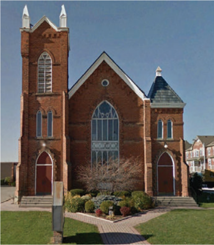
Woodbridge United Church. (Image Credit: Google Earth)
