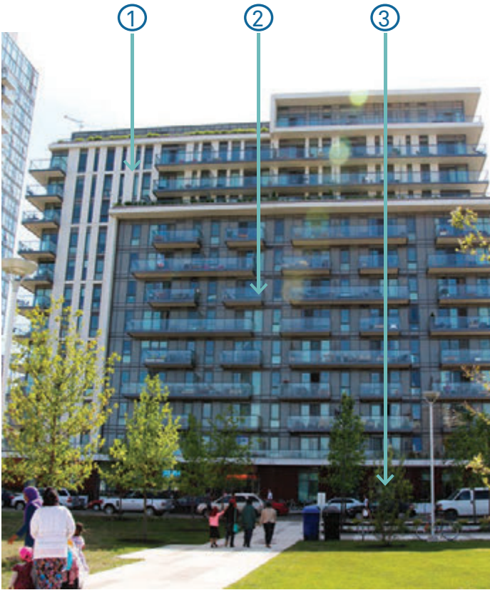
Distinct materials are used to create horizontal and vertical building components. (260 Sackville Street. Image Credit: Brook McIlroy)
