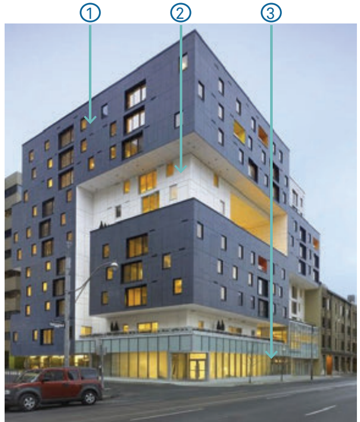
Significant glazing at the ground levels should be balanced with other materials on the upper levels. (Image Credit: 60 Richmond Housing Co-op, Teeple Architects)
