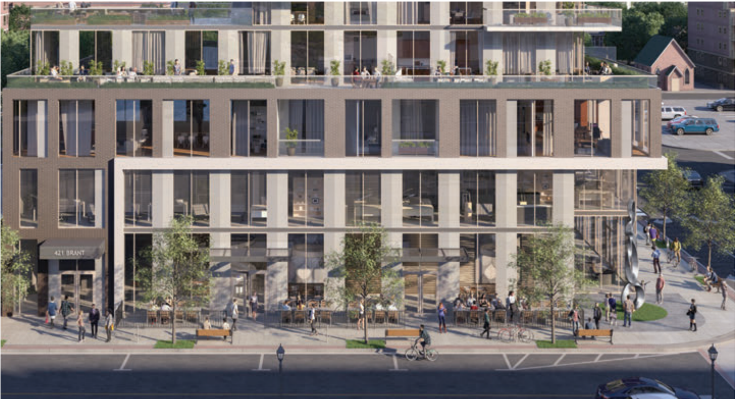
Large format retail uses in an urban format, including mixed-uses and articulated facade. (Image Credit: 421 Brant Street by Turner Fleischer Architects)
