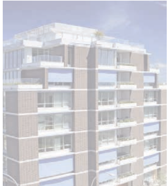
Well-screened rooftop mechanical equipment (Image: Dockside Green, Perkins+Will Architects)
