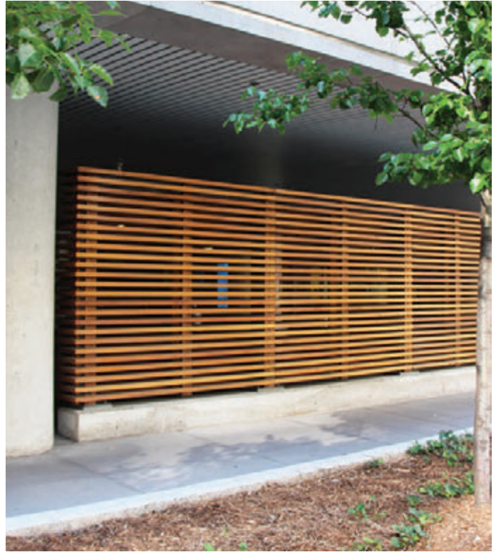
A wooden screen provides visibility as well as a visual buffer to a grade-level parking garage. (Image Credit: Brook McIlroy)
