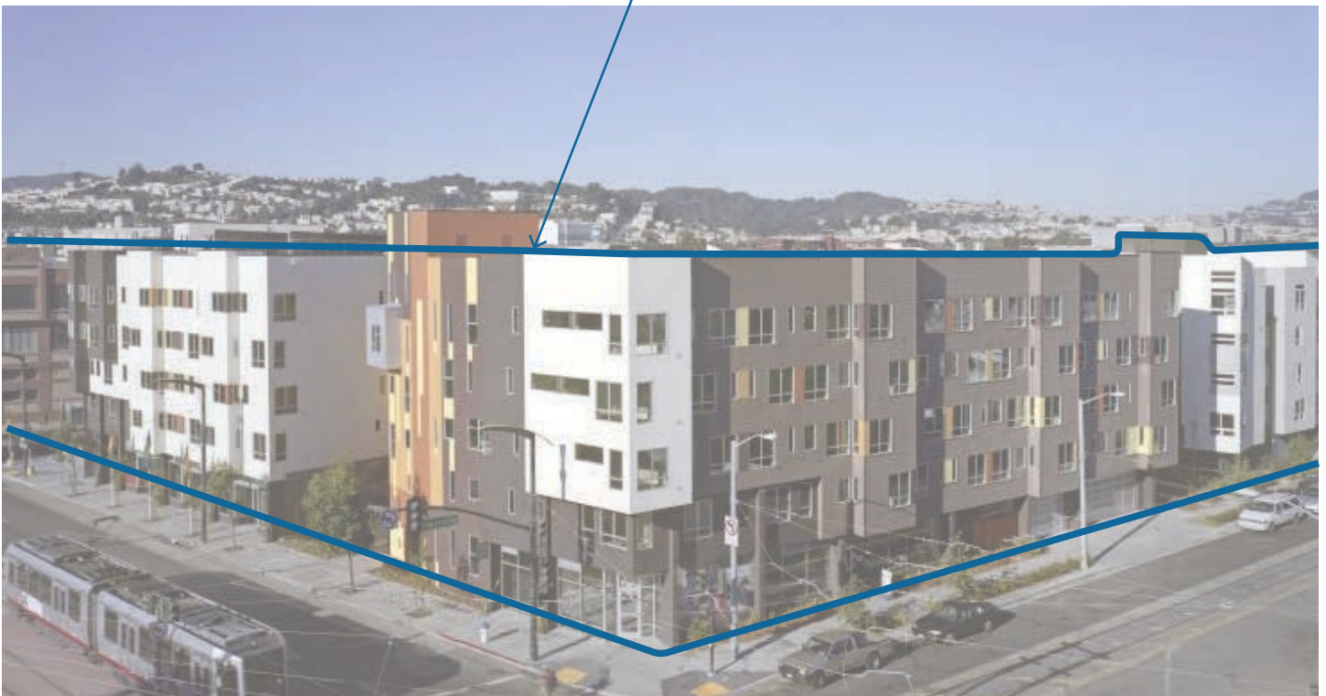
Low-Rise buildings should be designed to frame streets, open spaces and landscaped areas. (Image Credit: Armstrong Place Senior Housing, San Francisco, David Baker + Partners. Photo by Brian Rose)
