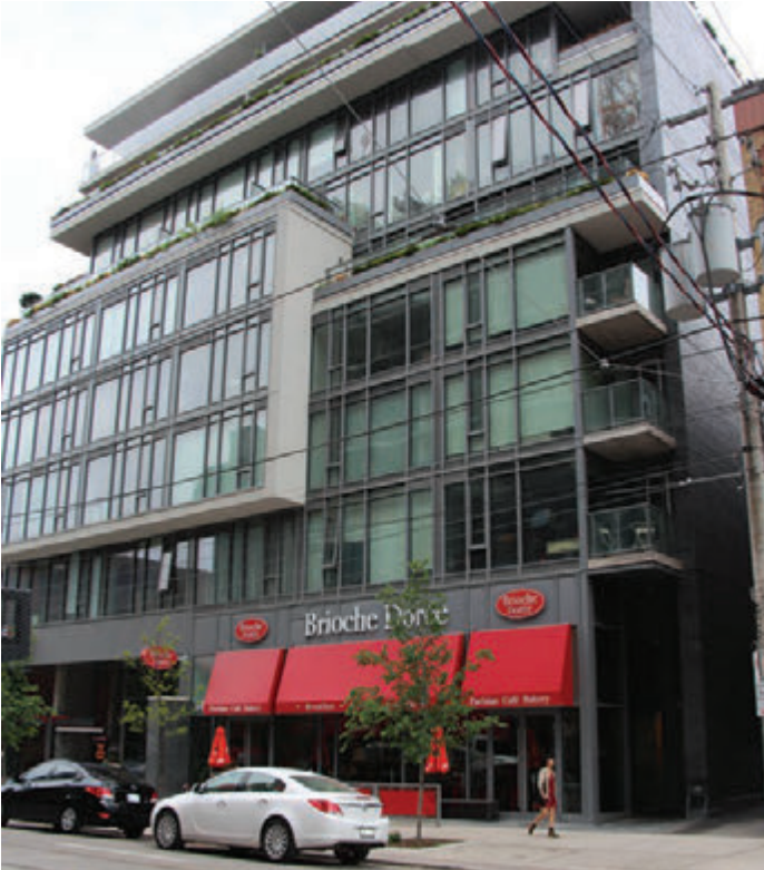
Building articulation helps to address downdrafts and other wind impacts on the pedestrian environment. (Image Credit: Brook McIlroy)
