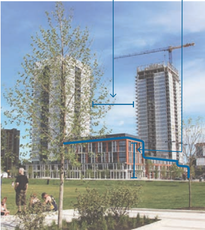
Adequate spacing between towers and building articulation, like lower-height podiums, can help to reduce downdrafts. (Image Credit: Brook McIlroy).
