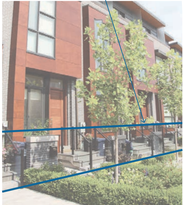
An enclosure for waste bins is integrated into the Townhouse design. (Image Credit: Brook McIlroy)
