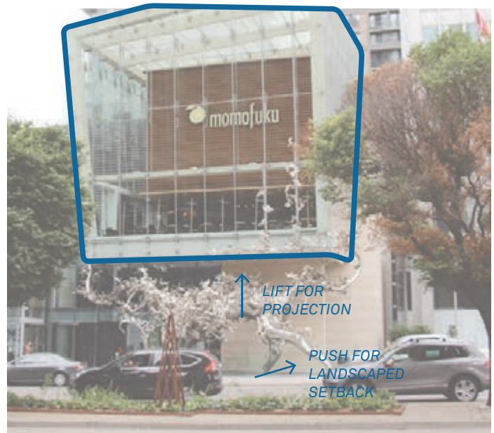
Projections above the Green Approach zone enhance articulation of the building envelope while providing space for an enhanced landscaped setback. (Image Credit: Brook McIlroy)
