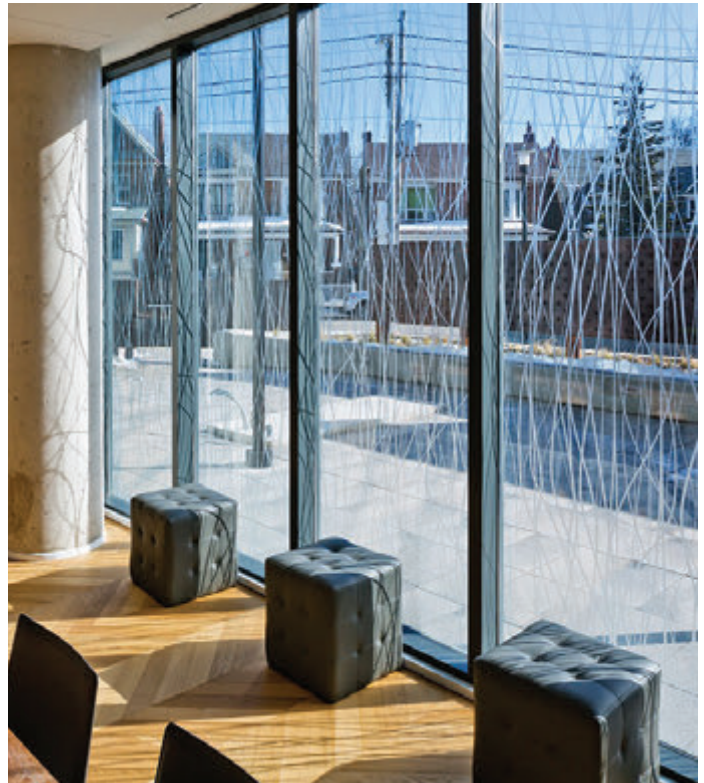
Treated glass to prevent bird strikes. (Image Credit: 60 Howard Park Ave, Toronto, RAW Design. Photo courtesy of Walker Textures)
