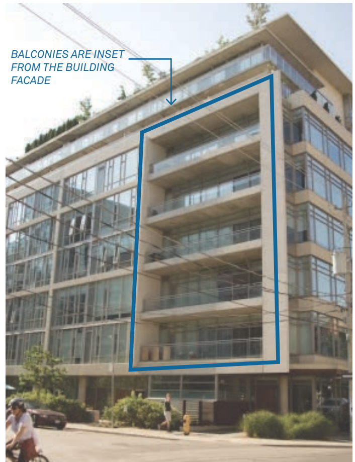
Inset balconies reduce the visual bulk of the building and provide interest to building massing. (66 Portland Street, . Image Credit: truelofts.ca)
