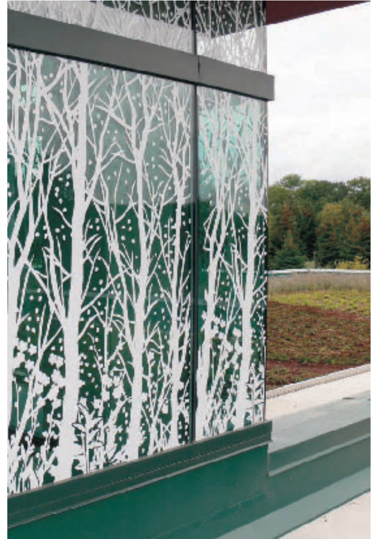
Externally-applied patterned decals can create sufficient visual markers for the glass to be perceived by birds Photo: Allan Turner
