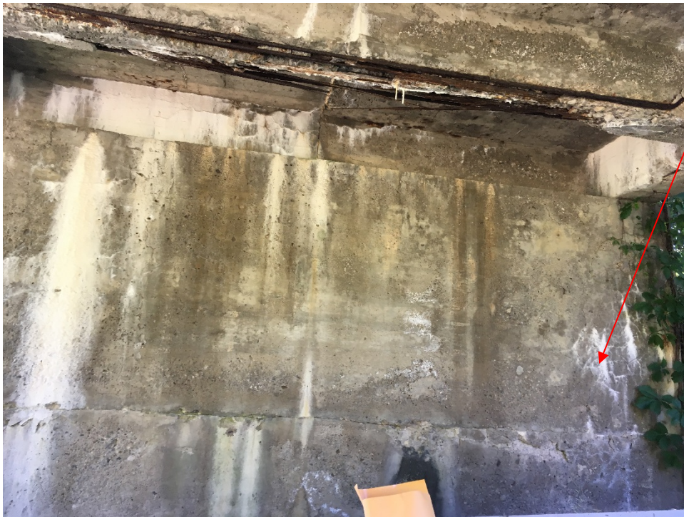
East abutment face from west
