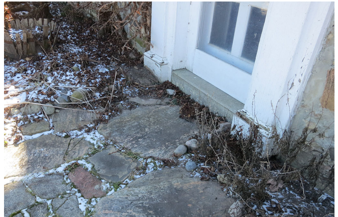
WCH - 14 North-east entrance paving
