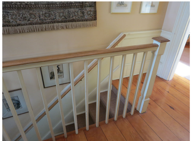
WCH-39 South landing stairs
