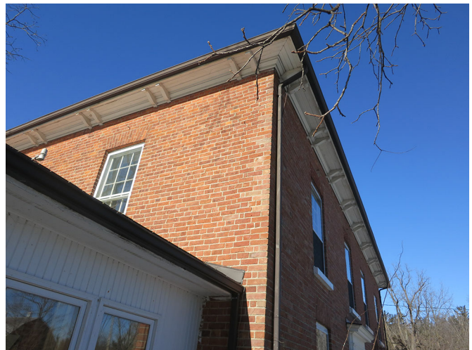
WCH - 10 Roof cornice and brackets
