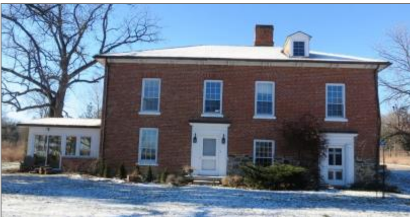
Figure 3-12 William Cook House Principal Facade
