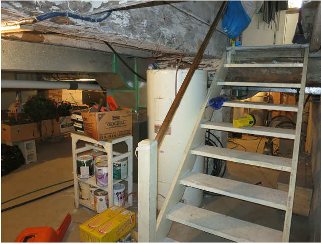
WCH-72 Basement stairs
