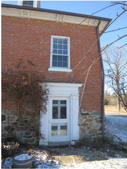
WCH - 13 North-east entrance
