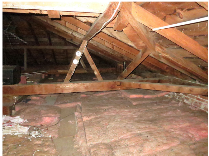
WCH-69 Attic timber frame
