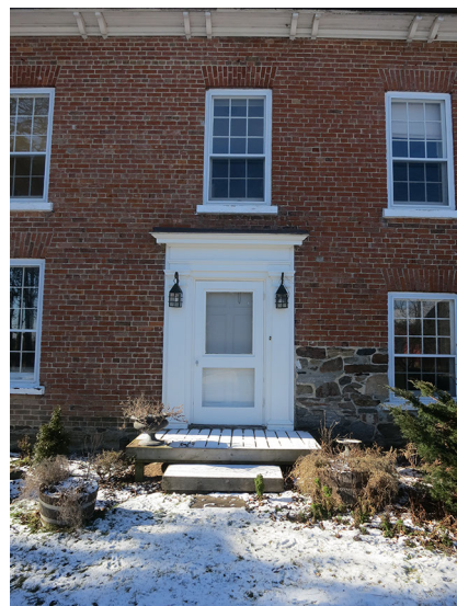
WCH - 12 South-east entrance
