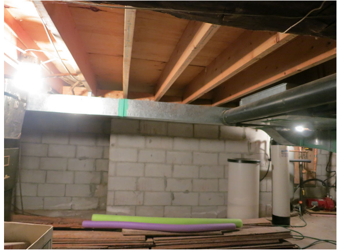
WCH-73 Basement new walls & joists
