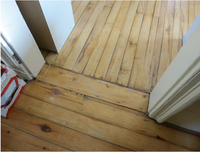
VKH-42 Hall to kitchen floor
