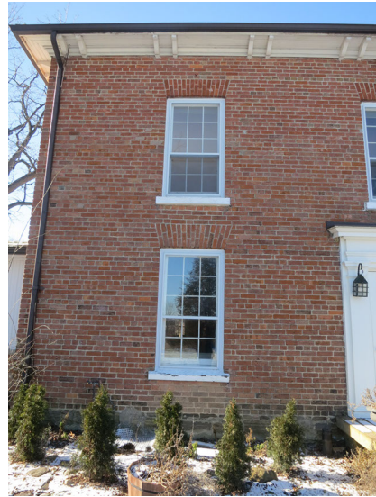
WCH - 08 East Elevation windows
