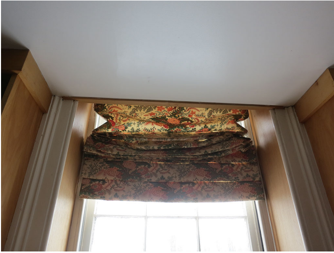
WCH-31 Kitchen ceiling
