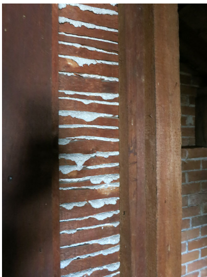
WCH-70 Attic split lathe
