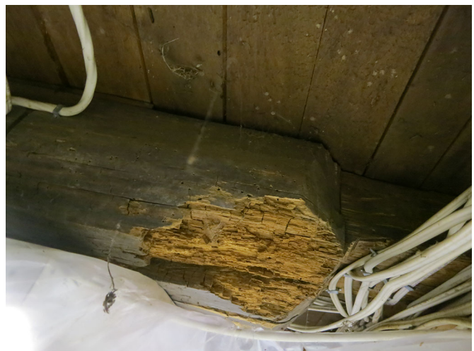
VKH-71 Basement floor beam
