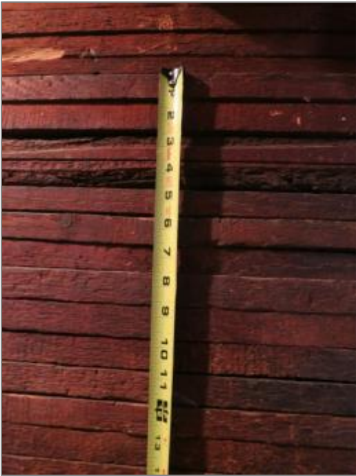
Figure 3-16 Valentine Keffer House Plank-on-Plank Construction detail
