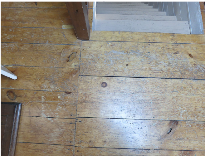
VKH-50 Upstairs hall floor
