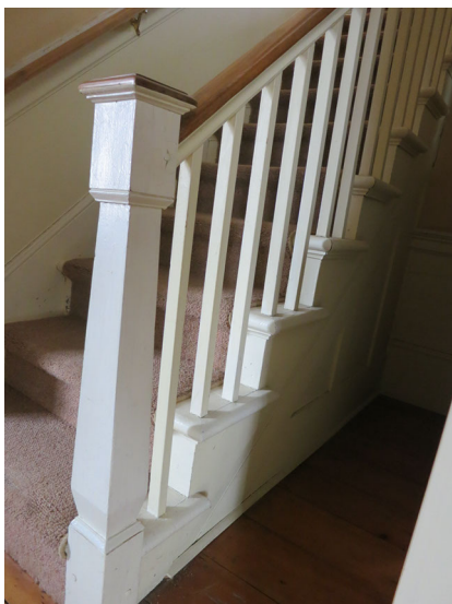
WCH-05 Front Hall stairs
