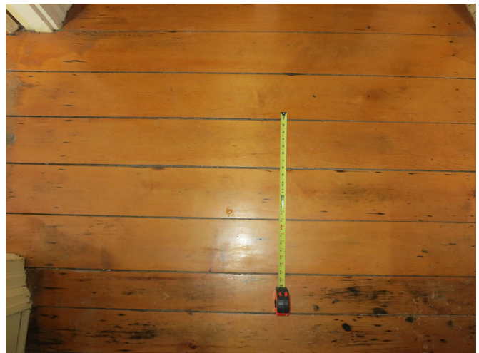
WCH-06 Front Hall floor
