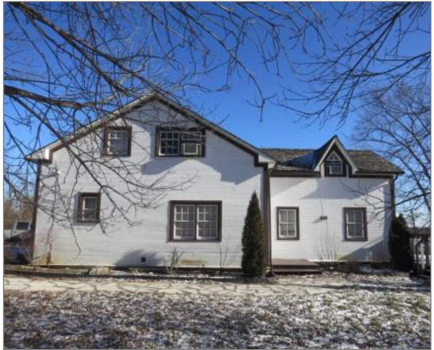
Figure 3-17: Valentine Keffer House Original (left) and Addition (right)
