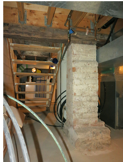
WCH-75 Basement brick support
