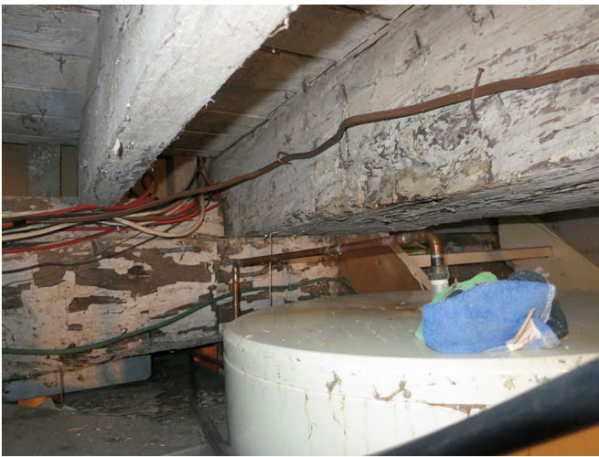
WCH-74 Basement old beams
