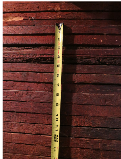
VKH-35 Stacked plank construction
