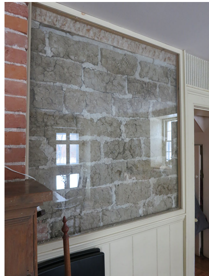
WCH-22 DR mud brick wall
