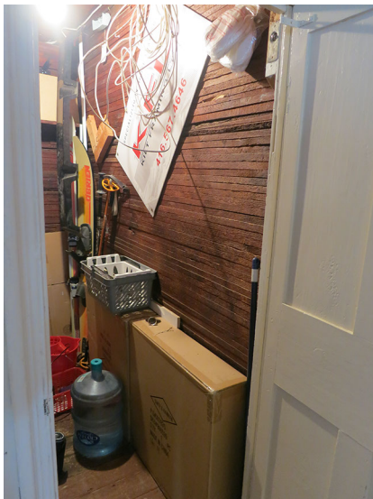
VKH-34 Stacked plank construction
