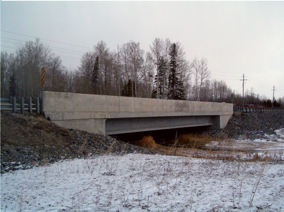
Photo 10 Example of Concrete Box Girder Bridge
