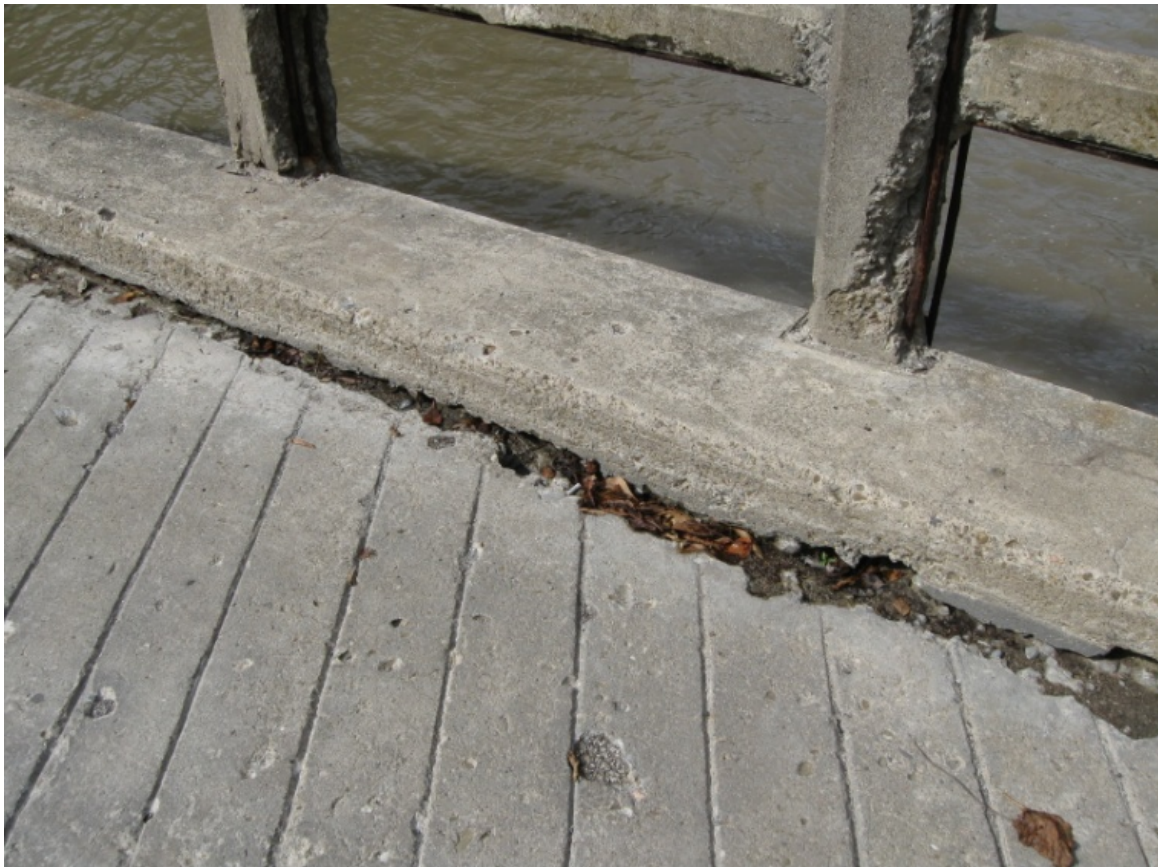
Photo 2 Curb on Deck
