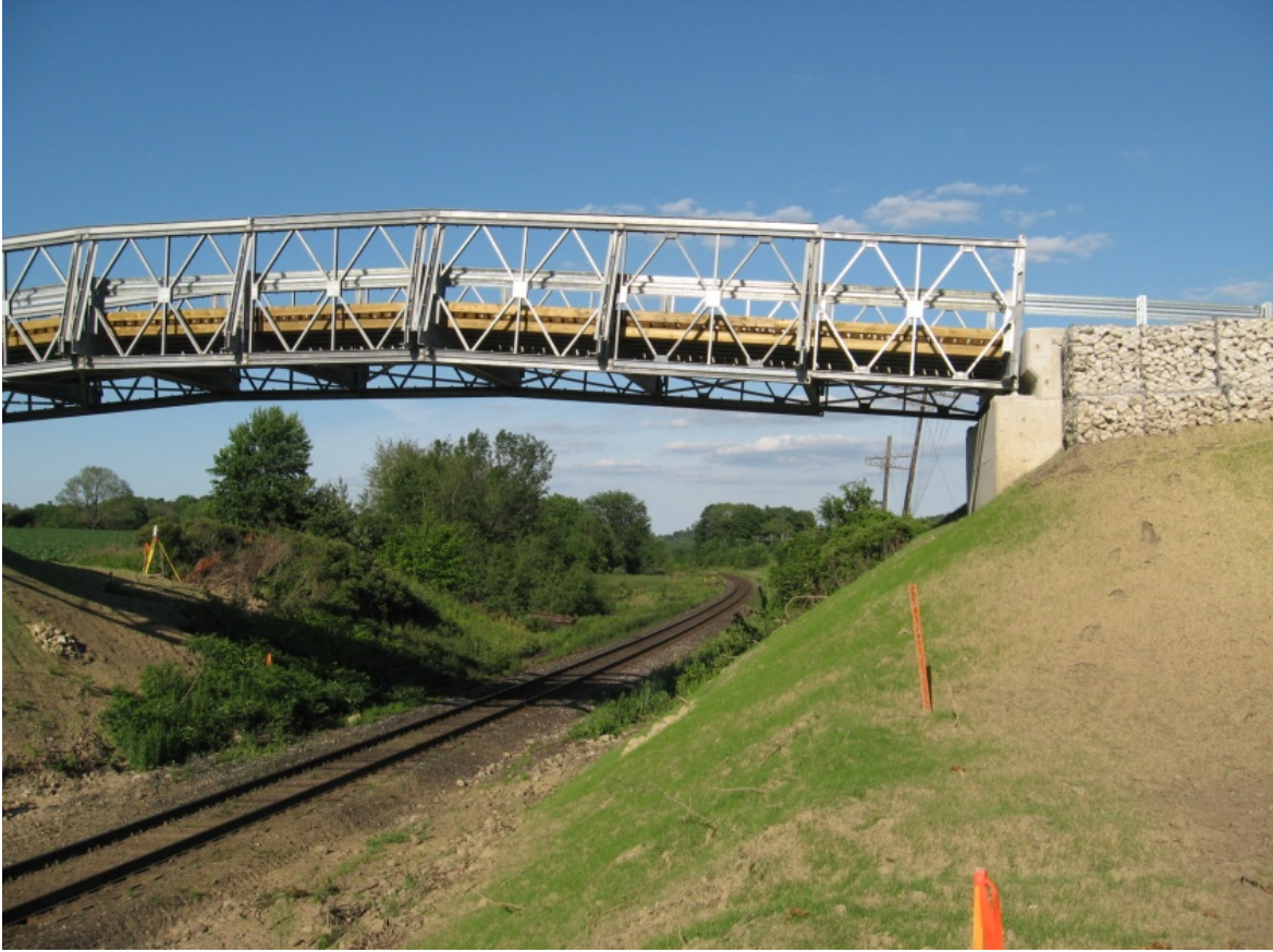
Photo 11 Example of Modular Bridge
