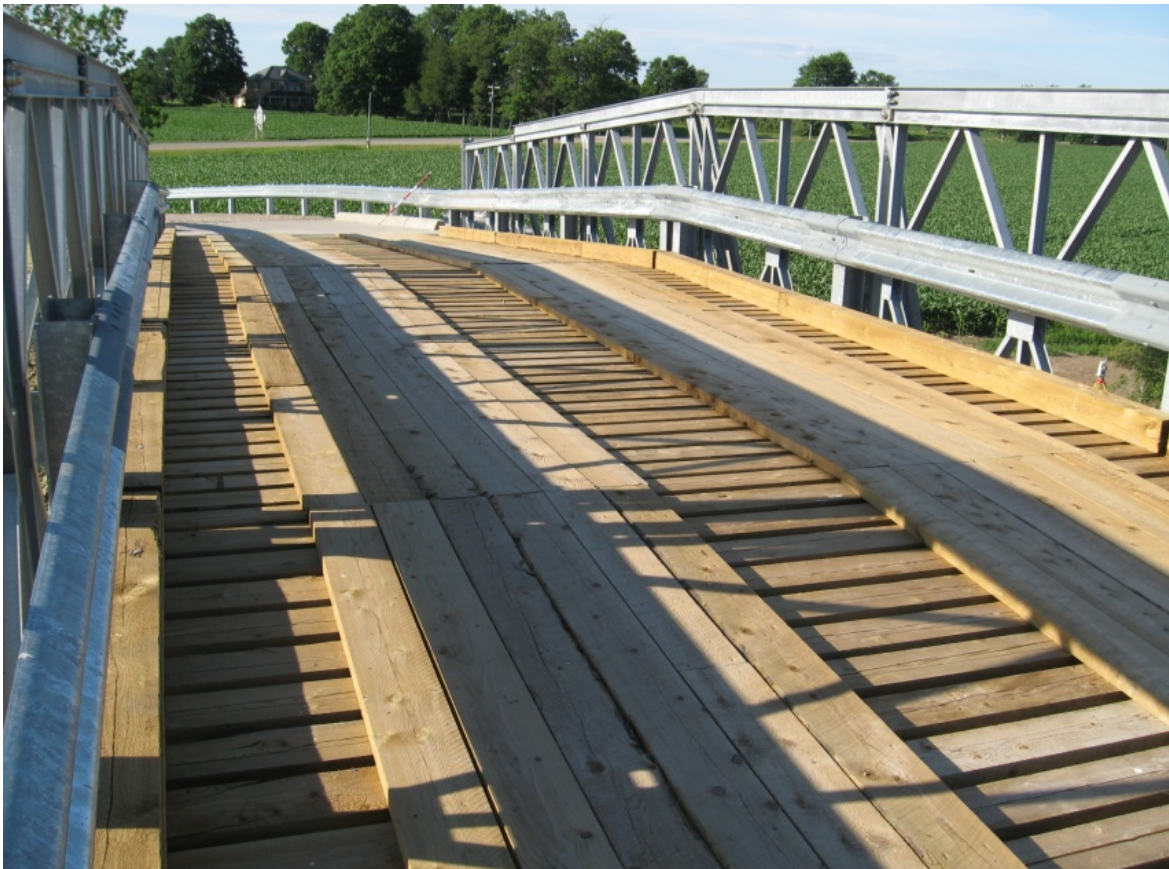
Photo 12 Close up of wooden deck, modular bridge
