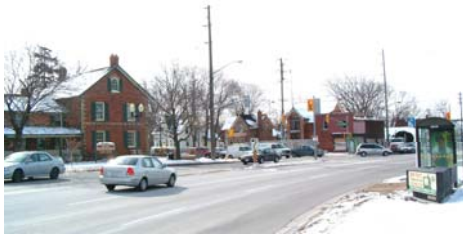
Rear flank of Beaverbrook House at the corner of Major Mackenzie Drive.
