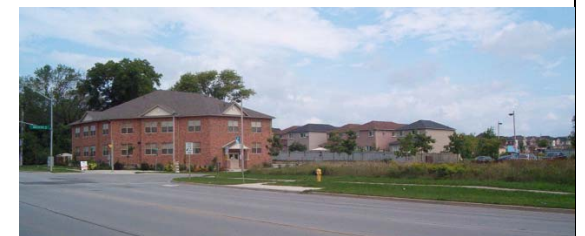
Looking over the corner of 10175 to the recent building at 10195.
