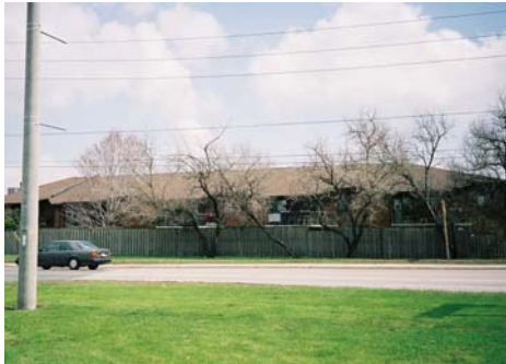
2185. Oriented to its parking lot, it makes a hole in the streetscape.
