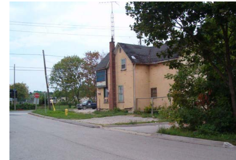
The rear flank of 2291 Major Mackenzie Drive sits at the north end of the street.
