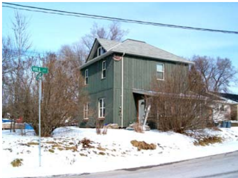
No 2 Hill Street. A four square house, unusual in that it was originally clad in stucco. Board and batten siding is a recent renovation.
