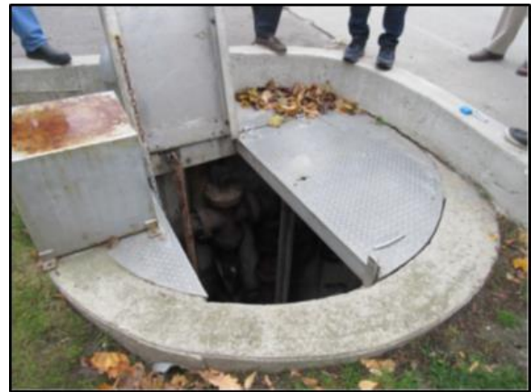
Pumping Station Maintenance
