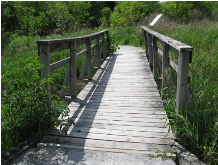
Keffer Marsh Bridge, Thornhill (Don River)
