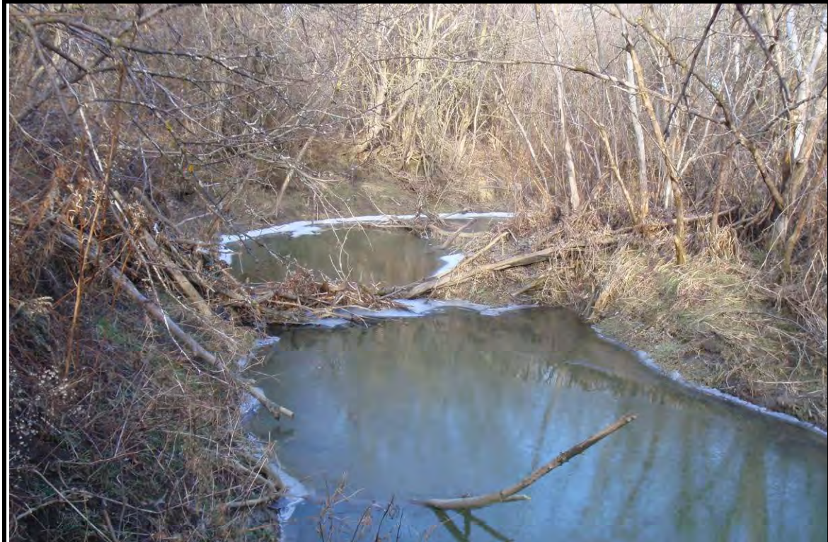
PHOTOGRAPH NO.: B11 FROM: LOOKING: Upstream COMMENT: Reach West 3 bank erosion
